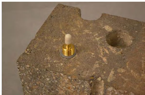
Figure 3. Installed VAPOR PIN®
