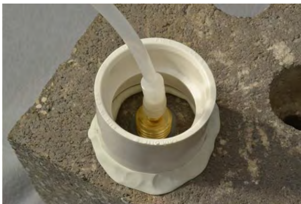
Figure 6. Water dam used for leak detection
