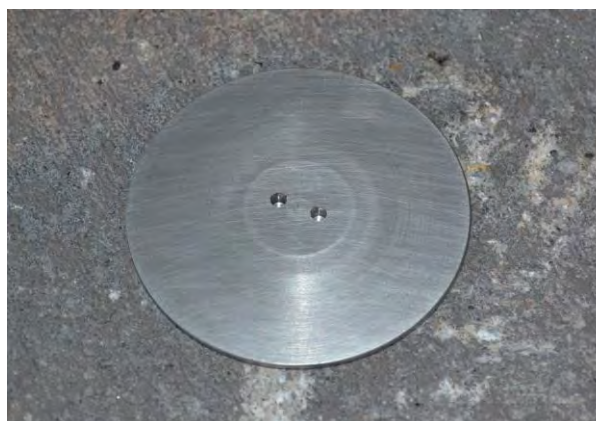
Figure 4. Secure Cover Installed
